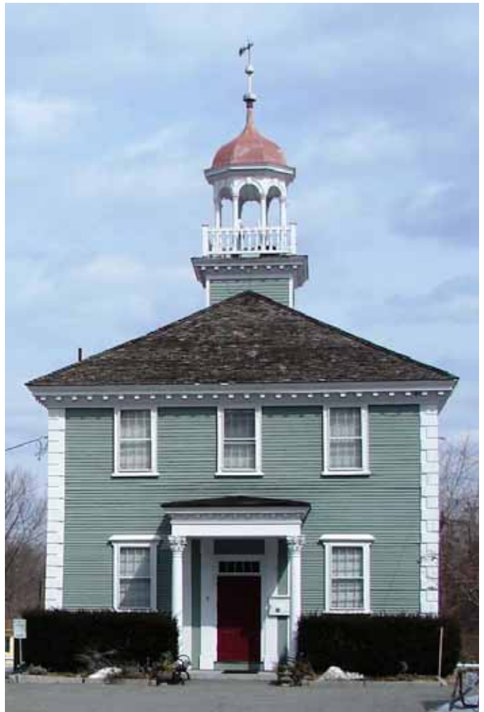
The Westford Museum in Westford, MA, is a late-eighteenth-century academy building that did duty as a firehouse throughout much of the twentieth century before being converted in 1985 to a museum facility for the Westford Historical Society.
