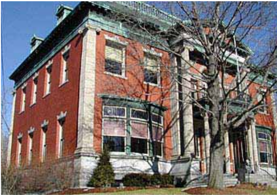
The Clinton (MA) Historical Society's handsome home for well over a century, a 1904 Beaux Arts building known as the Holder Memorial, offers a surprising and beautiful two-story interior hall (below). In 2014, the society celebrated its 120 th anniversary.
